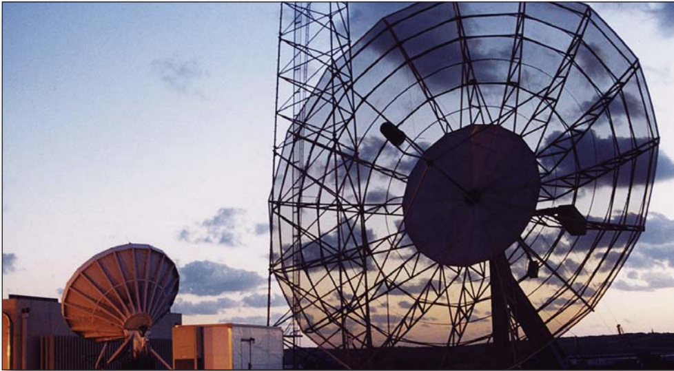
Fast Speed communications tower and antenna.
